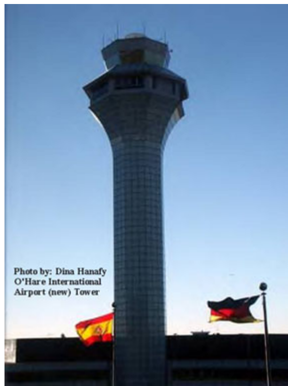
Figure 7. New O'Hare Airport Control Tower
